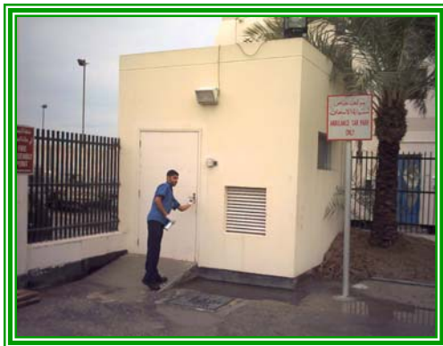
i) Secured Storage room for Hazard waste
